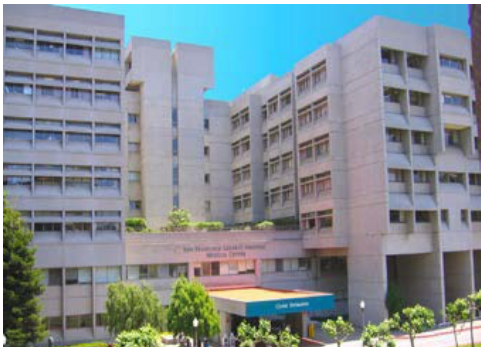
Existing Main Hospital, Building 5 at the Potrero Campus
