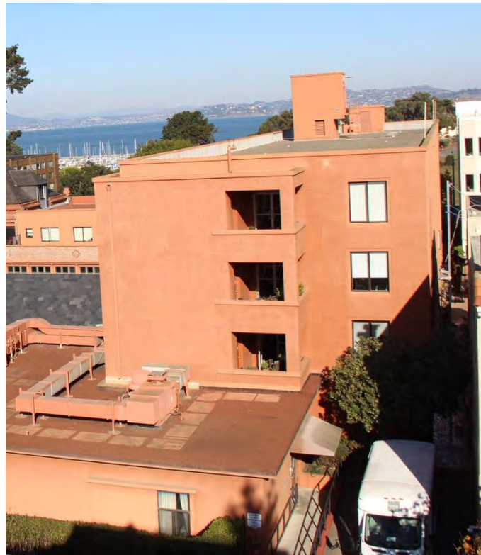
Figure 30. Residential wing of the Perry Building; view from building on Francisco Street.
