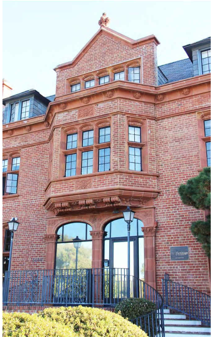
Figure 19. Main entrance with oriel above.
