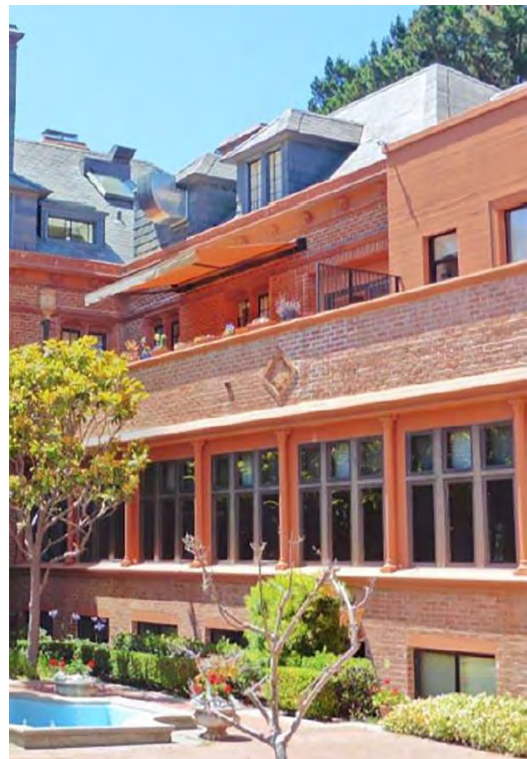
Figure 26. Juncture of (north) rear wing of Morgan Building and 1957 Perry Building. Source: Page & Turnbull
