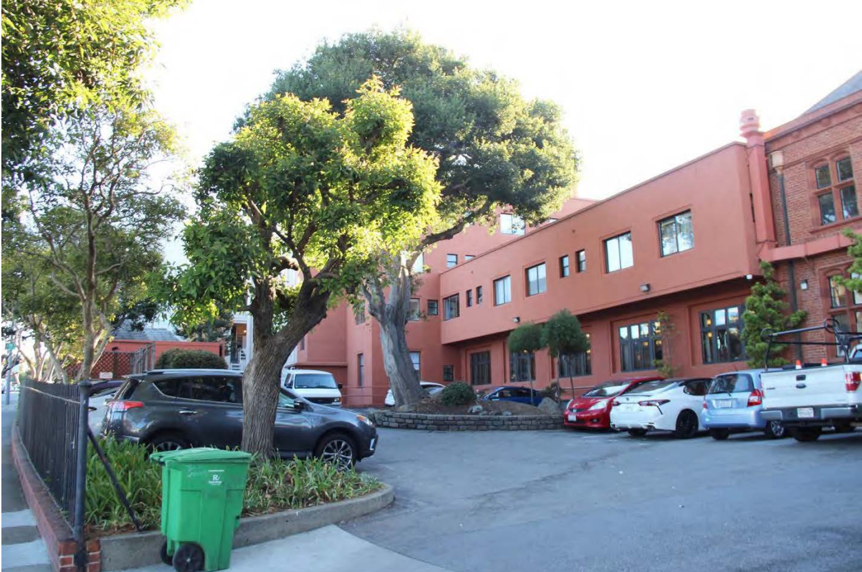
Figure 14. Parking lot at north side of property.
