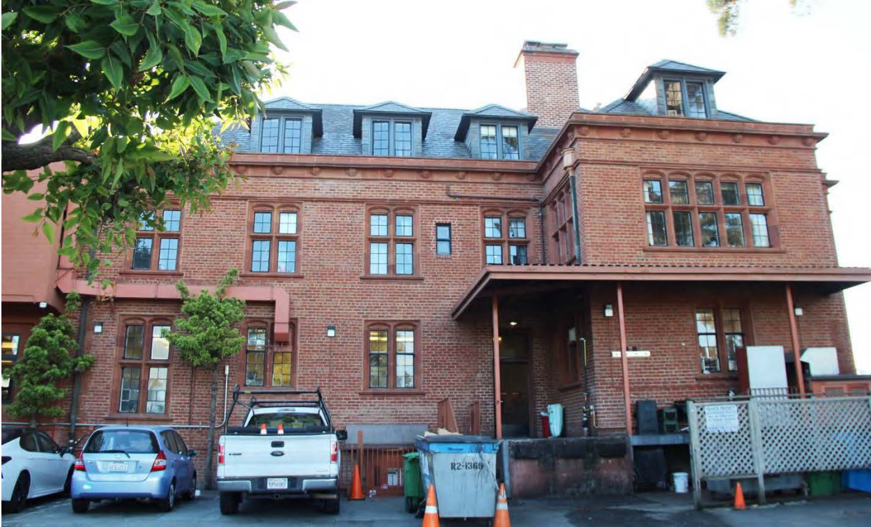
Figure 21. North (secondary) façade of the Morgan Building.
