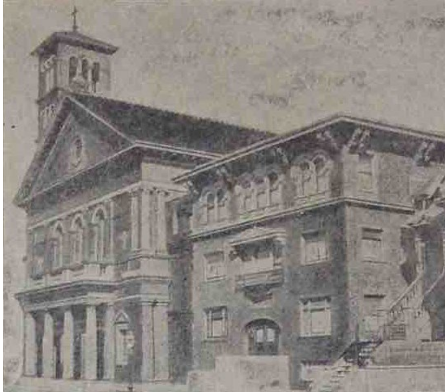
FIGURE 58. CHURCH AND RECTORY SHOWING ORIGINAL DOOR AND WINDOW TREATMENT ON FIRST AND SECOND STORIES. SOURCE: CATHOLIC MONITOR, OCTOBER 2, 1920
