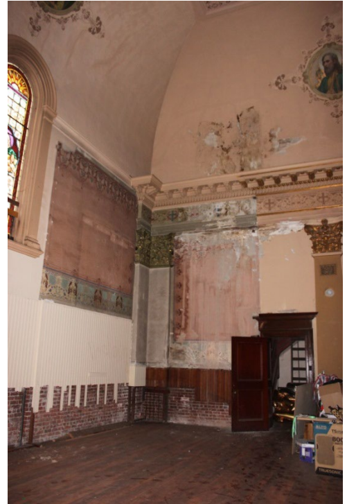
FIGURE 21: CHURCH: CHOIR LOFT, NORTHWEST CORNER AND DOOR TO STAIRS, SHOWING FINISH MATERIALS AND DECORATIVE TREATMENTS, 2016.
