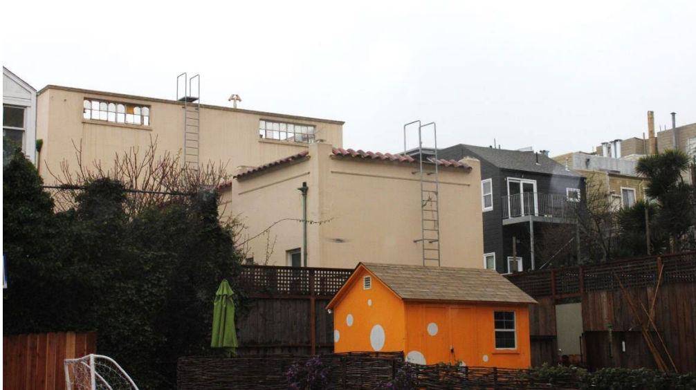
FIGURE 51. CONVENT: REAR (NORTH) ELEVATIONS OF CHAPEL ELL AND MAIN BLOCK, 2016.
