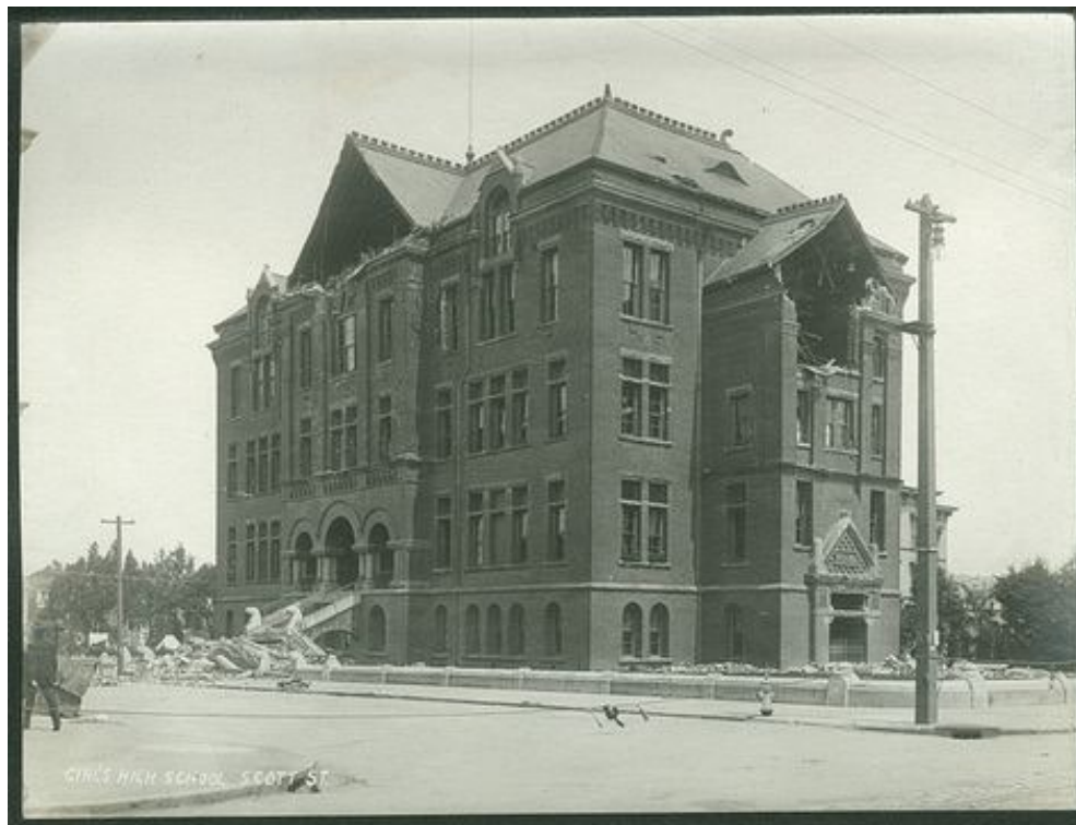
FIGURE 82. WELSH'S GIRLS HIGH SCHOOL AFTER DAMAGE IN THE 1906 EARTHQUAKE. SOURCE: DELGOYER LIBRARY, SOUTHERN METHODIST UNIVERSITY
