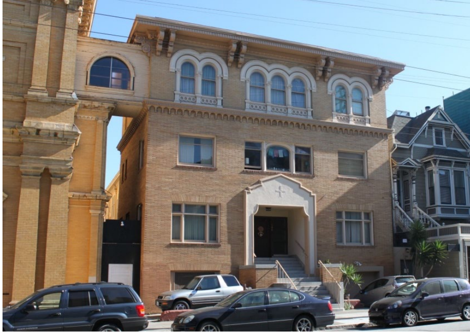
FIGURE 38. RECTORY: MAIN (WEST) ELEVATION FROM FILLMORE STREET, 2015.
