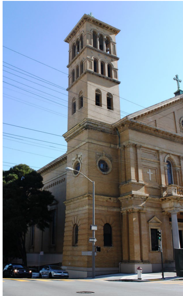
FIGURE 7. CHURCH: CAMPANILE, LOOKING SOUTHEAST FROM FILLMORE ST., 2015.
