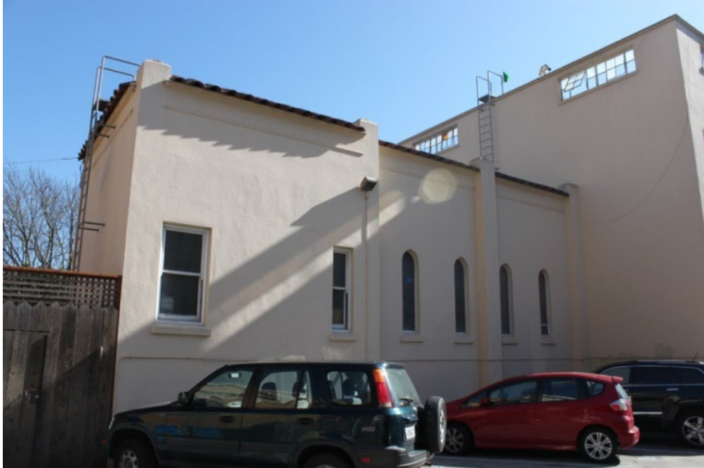
FIGURE 50. CONVENT, CHAPEL WING, LOOKING SOUTHEAST FROM PARKING AREA OF OAK ST., 2015.
