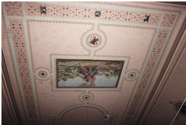
FIGURE 29. CHURCH: NAVE, WEST PORTION OF PAINTED CEILING, 2016.
