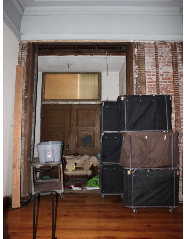
FIGURE 17 (RIGHT). CHURCH: BAPTISTRY SHOWING PARTIAL REMOVAL OF WALLS AND DOOR TO INTERIOR ALLEY, 2016.
