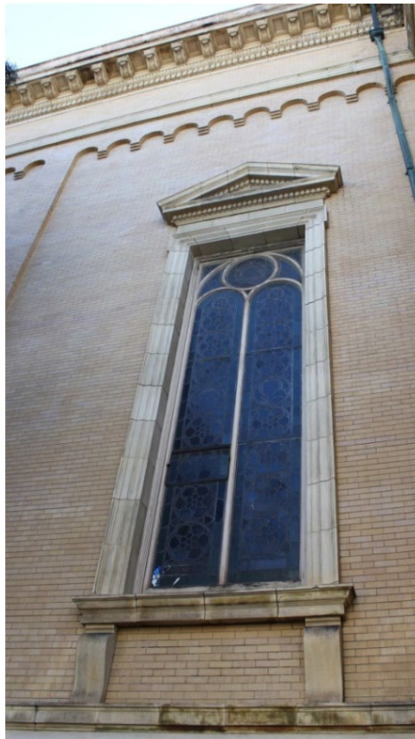
FIGURE 9. CHURCH: NORTH ELEVATION, DETAIL OF WINDOW, LOMBARDY BAND, AND CORNICE, 2015.
