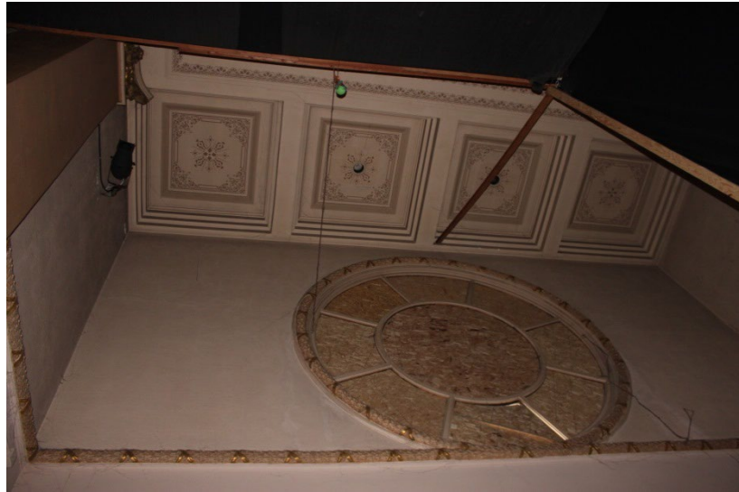
FIGURE 30: CHURCH: NORTH TRANSEPT SHOWING DECORATIVE DETAILING, 2016.
