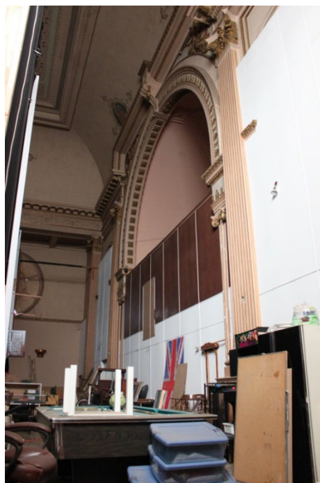
FIGURE 32. CHURCH: SANCTUARY SHOWING SEALED ALTAR NICHES, 2016.
