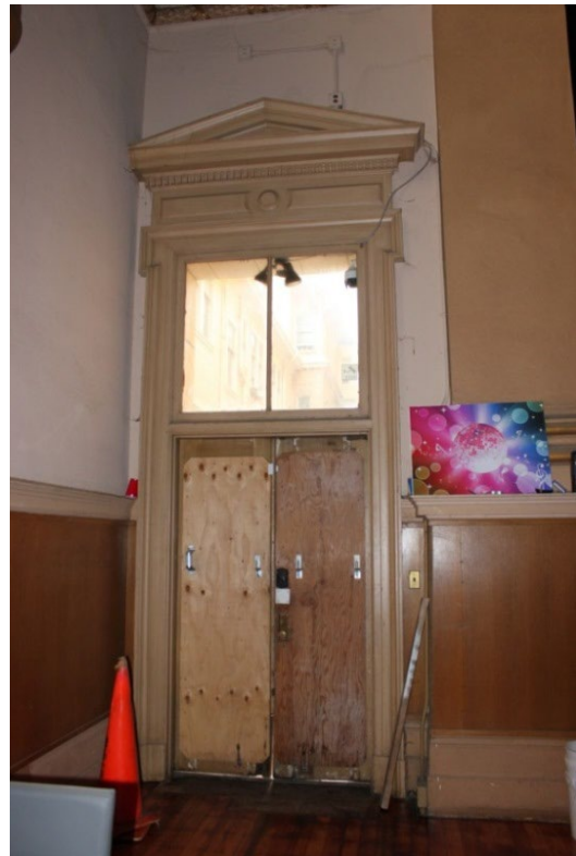
FIGURE 31: CHURCH: NAVE, SOUTH TRANSEPT ENTRY TO ALLEY, 2016.
