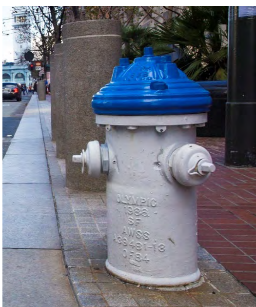
Figure 4. Example High-Pressure Fire Hydrant
